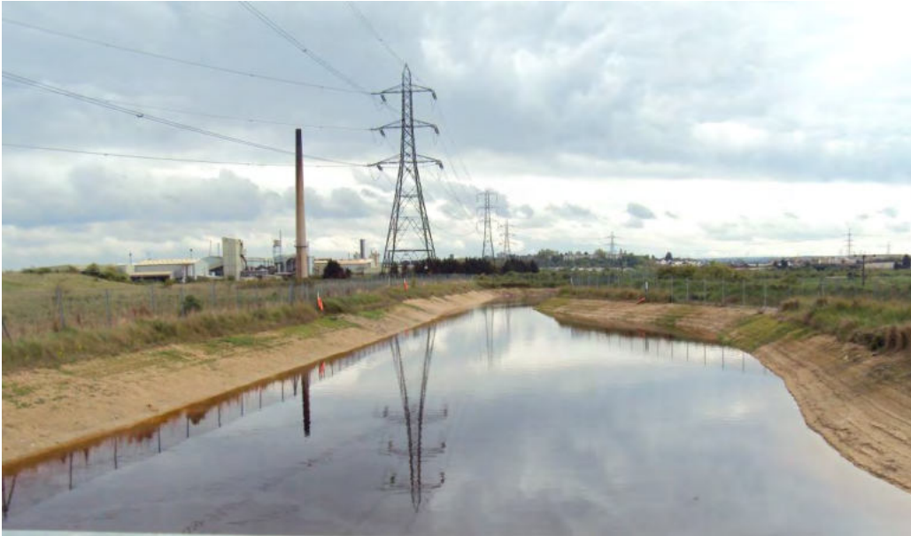
Figure A3 Pond with steep-sided bare soil banks. The water is discoloured red/brown-possibly due to leachate contamination (P4)
