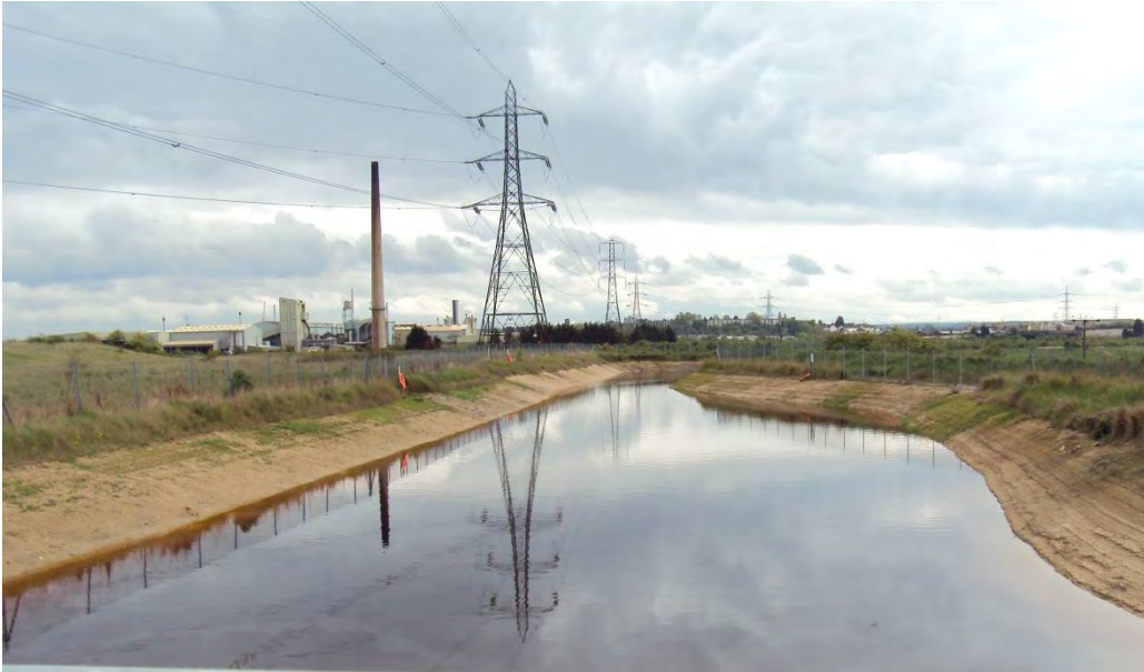
Figure A3 Pond with steep-sided bare soil banks. The water is discoloured red/brown-possibly due to leachate contamination (P4)
